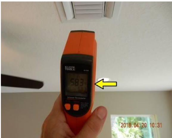
Supply Air Temperature: 58.3 Degrees F.
