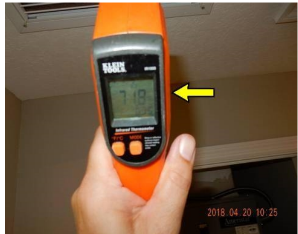
Return Air Temperature: 71.8 Degrees F.
